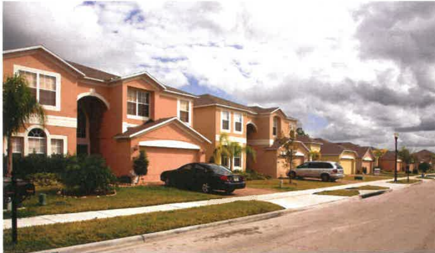
VIEW OF RESIDENTIAL STREET.
